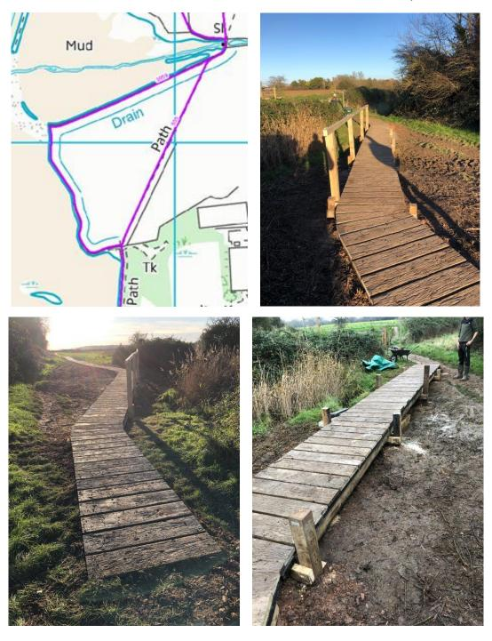
The boardwalk was installed as a potential short-term measure, pending the outcome of the Feasibility Study. The boardwalk can be moved, raised, or relocated at a later date if required.
