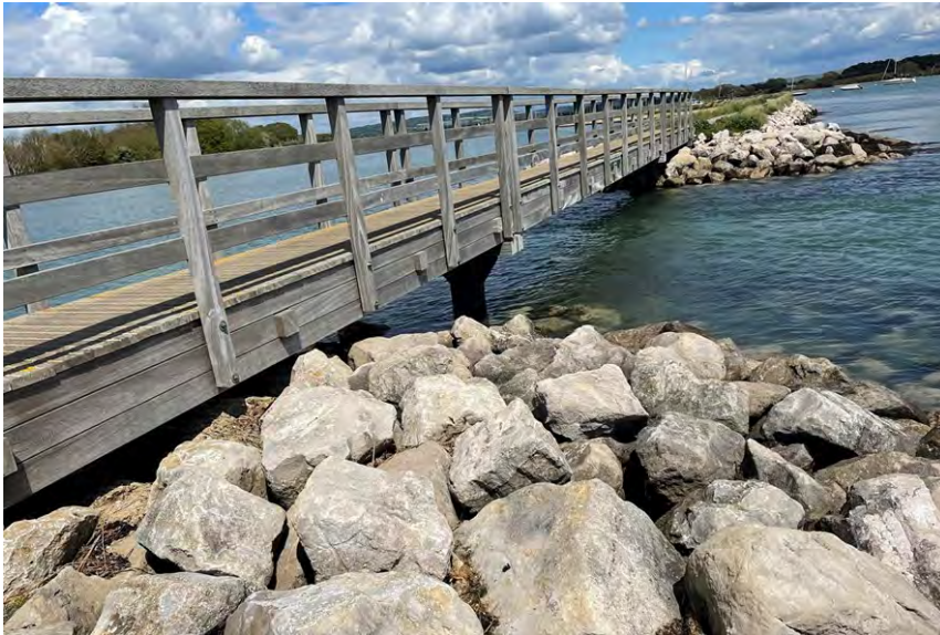
Figure 8-2 Bridge over one of the Cobnor Point managed realignment scheme breaches. Photograph taken 26 th May 2021 courtesy of Uwe Dornbusch
