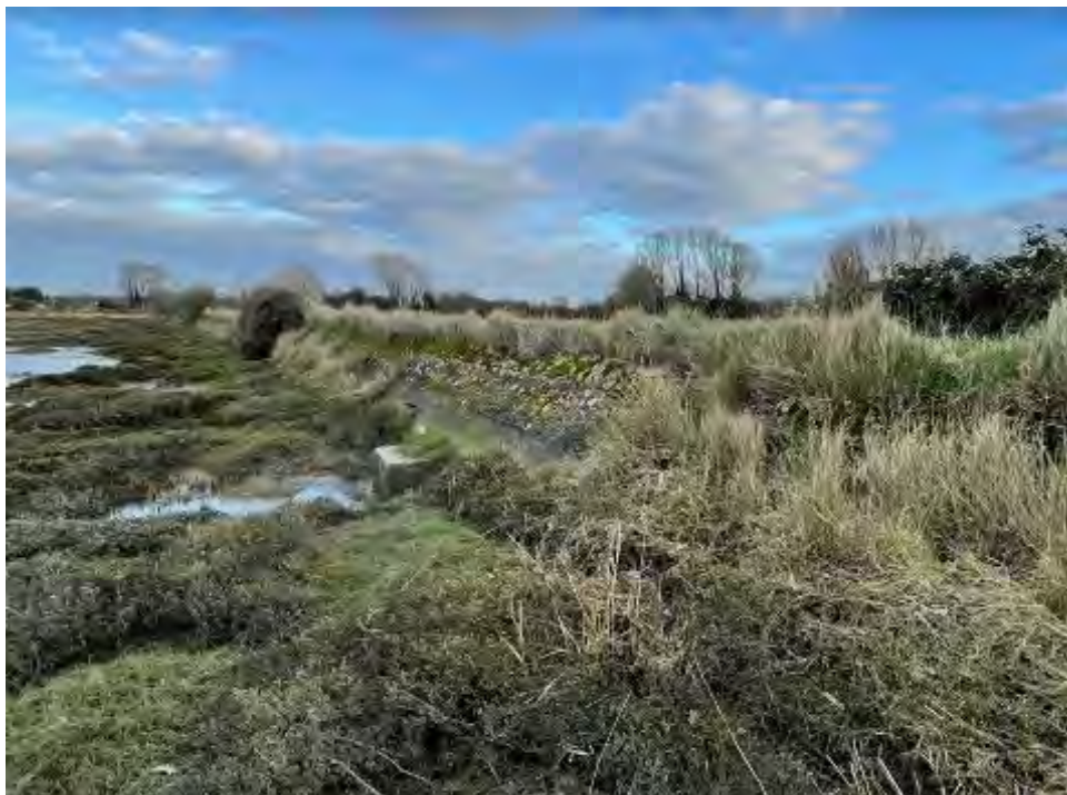
Figure 2-2 Embankment along the northern boundary of the site
