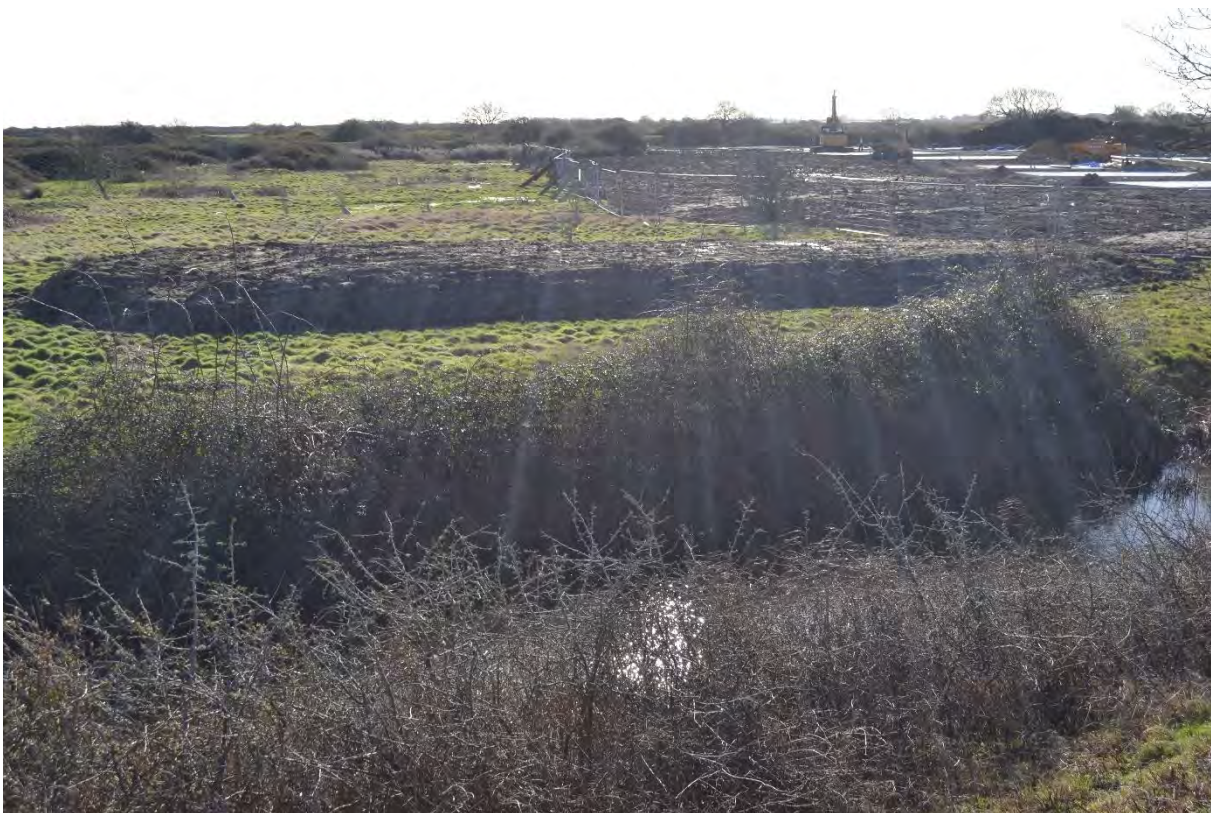
Figure 3.14. Construction of an extension of Mill Rythe Coastal Village across coastal grazing marsh to its east
