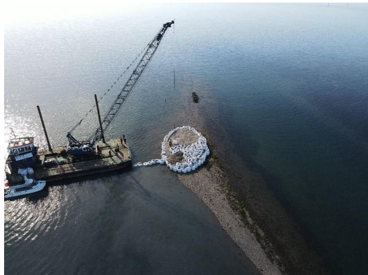
Stakes Island Shingle recharge
