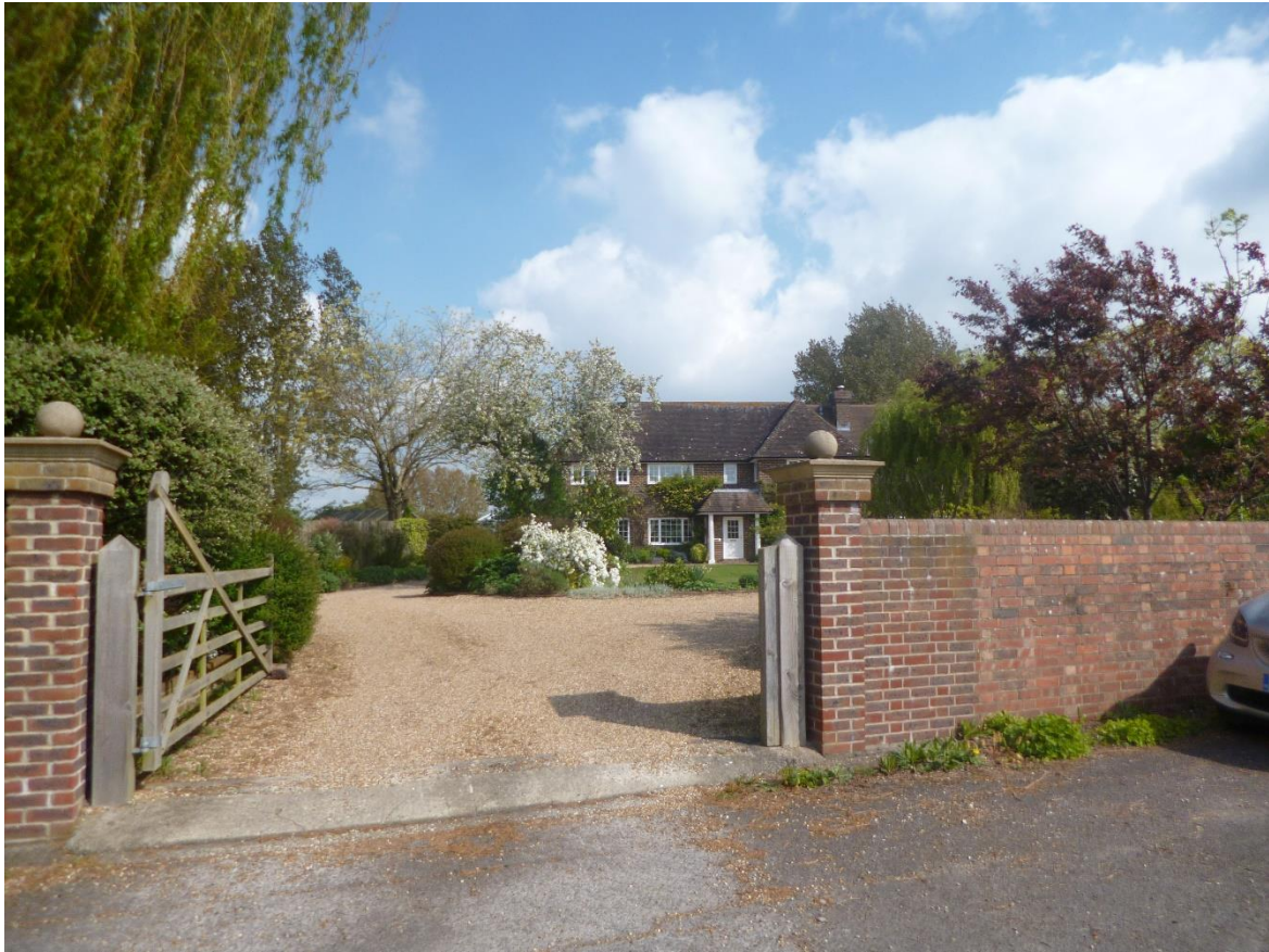
Above: Front of house as viewed from opposite driveway entrance
